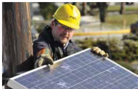
PSE&G lineman Ryan Lucas adjusts a solar panel. PHOTO: MARK LOVRETIN/PSEG
